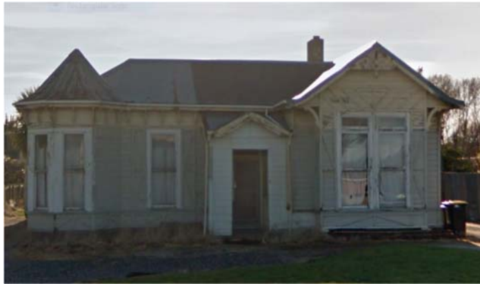
Taken prior to demolition in 2019/20
